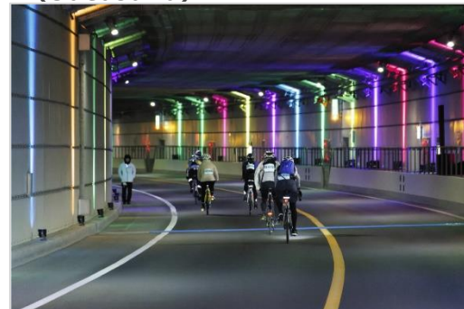
Tokyo Harbor Uminomori Tunnel (Outbound)
